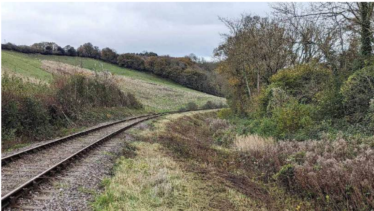
The line near Kentsford Farm Crossing after a visit from the Road Rail Vehicle and its flail attachment, in late autumn (27 th November 2024) Photo: Jake Genge
